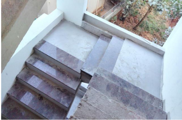
FIRE STAIR GRANITE WORK PROGRESSING
