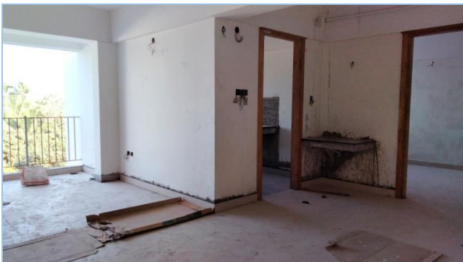
CARPENTRY WORK IN PROGRESS
