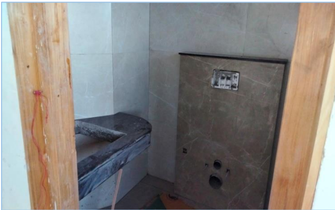
TILE WORK IN PROGRESS
